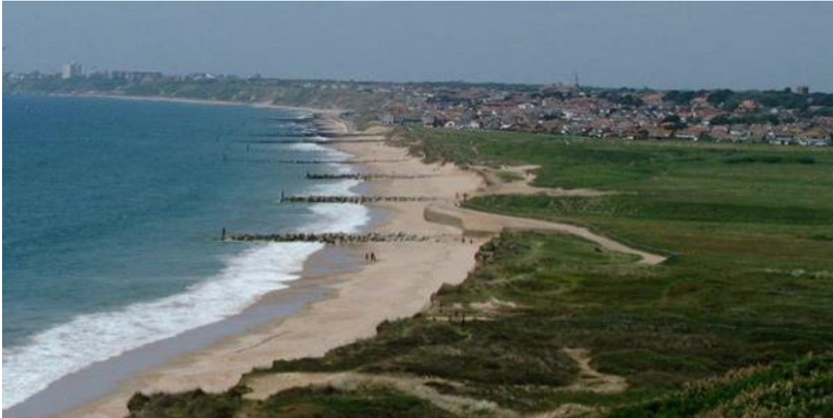
Figure 24: Rock groyne system (Source: CCO, 2018).
