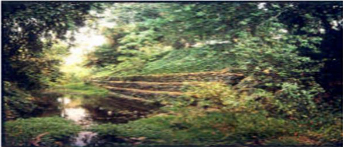
Figure 20: Gabion baskets installed for slope stabilization along a stream (Source: Freeman, 2000).
