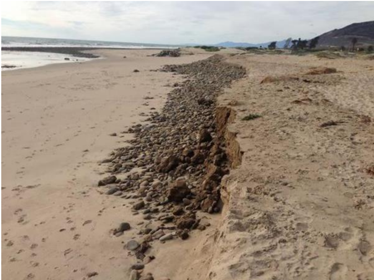
Figure 26: Cobble Berm Installed at Surfers' Point (Source: CRT, 2018).
