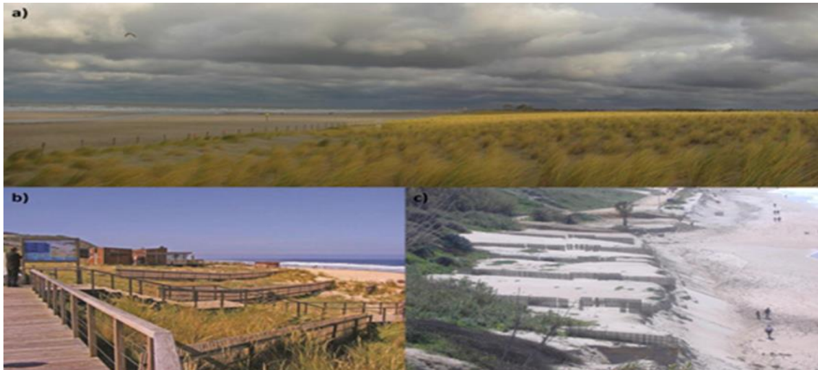
Figure 14: Example of dune stabilization by the use of planting, fencing and thatching at (a) Netherlands, (b) Portugal, (c) Spain (Source: Gracia et al., 2018).
